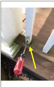
Wood softening on stiles rails. Repairs needed.
