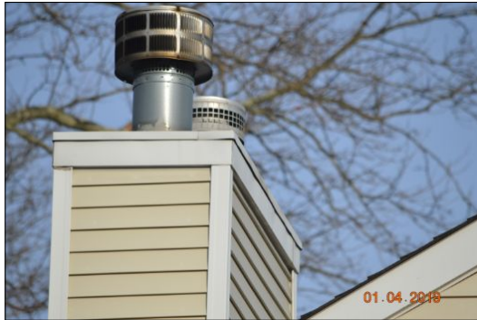
Chimney encase in siding
