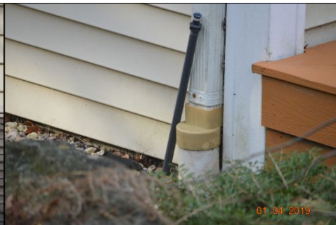
Some gutters drain under ground
