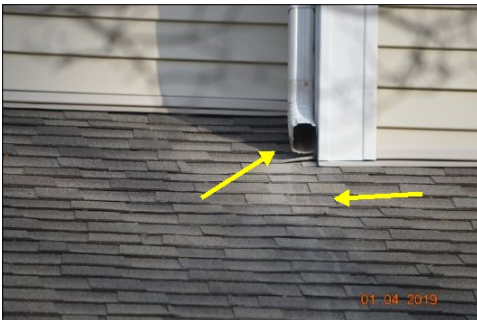
Upper gutter drains to roof
