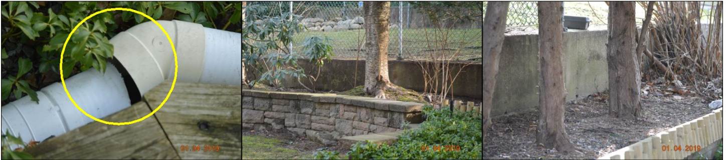
Damaged weeping pipe
