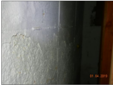
Efflorescence observed
