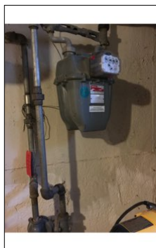
Located in front of basement
